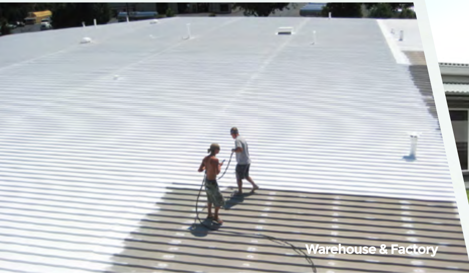
Restoration of Metal Roof
